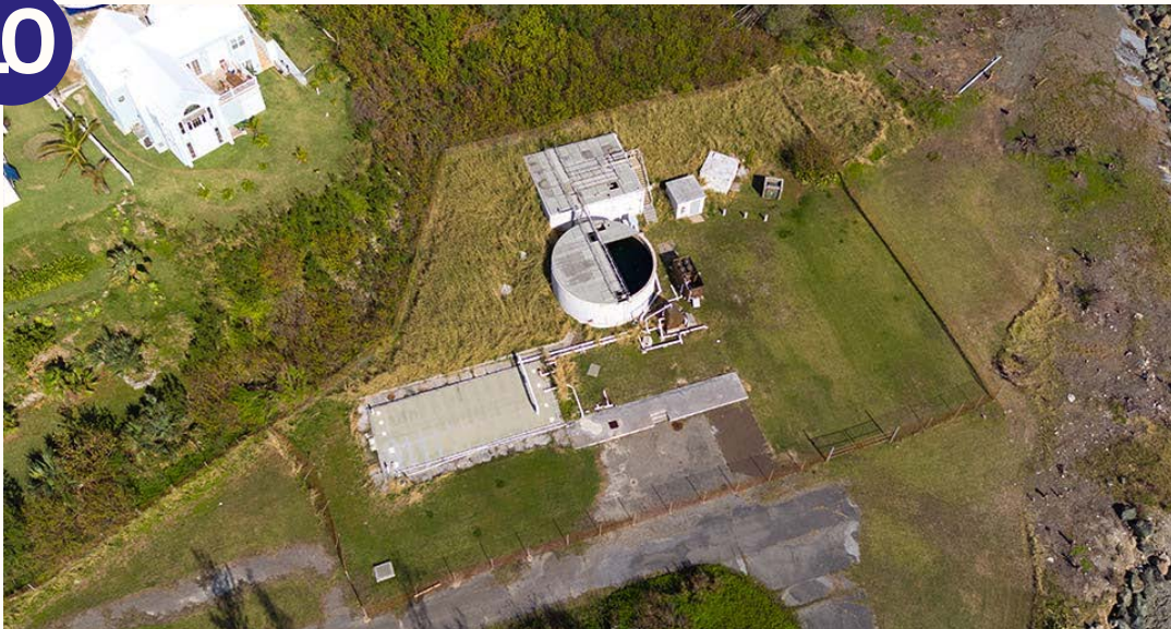
Old Sewage Plant area Approximately .5 acres Zoned - Mixed Use
